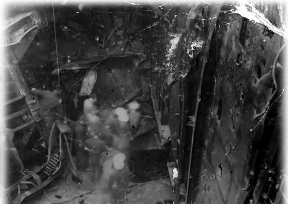
Damage to the aft aircraft lift
