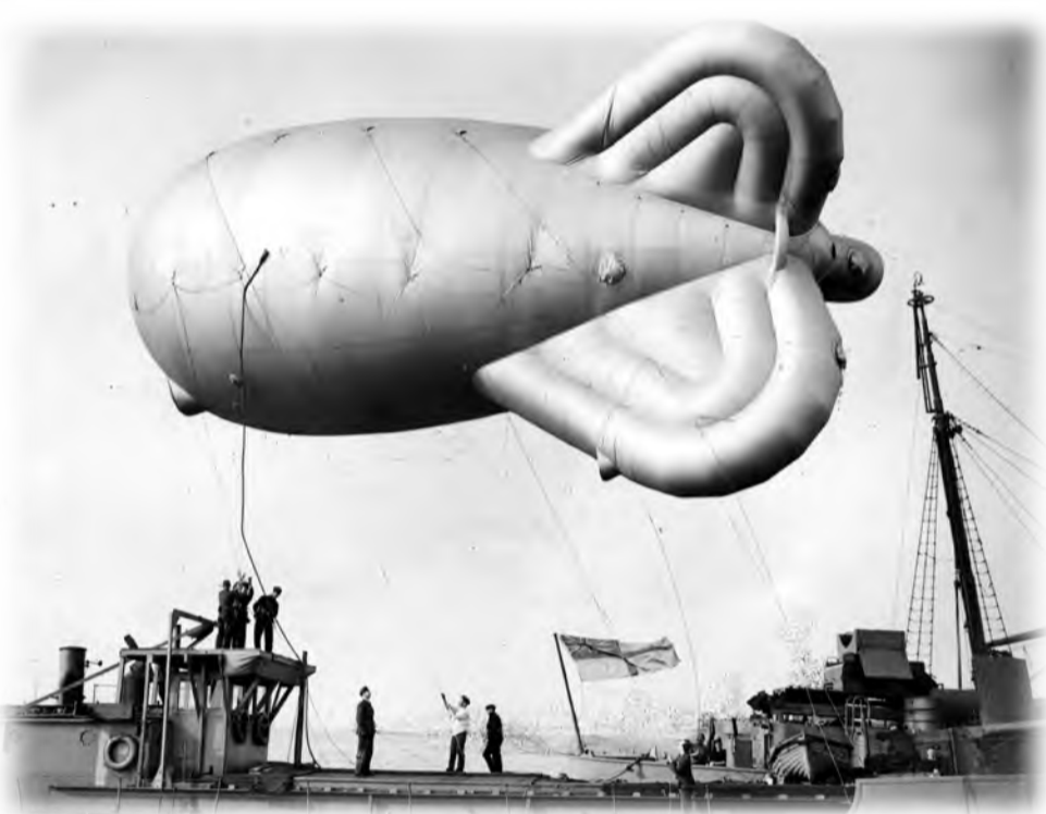
Barrage Balloon being raised aboard a vessel at Sheerness
