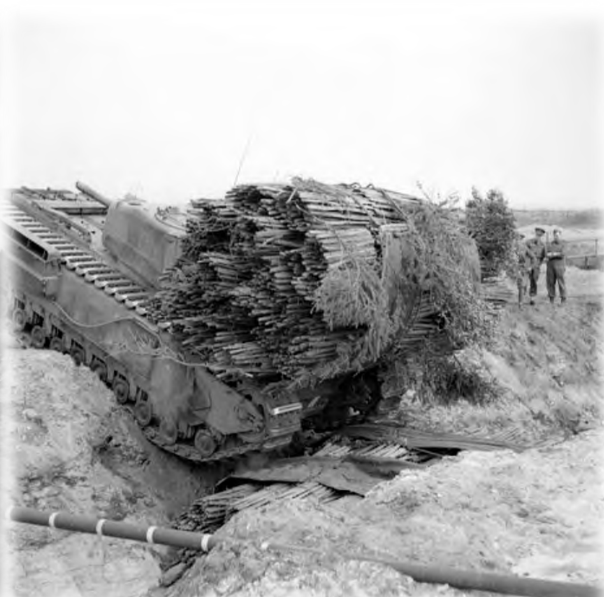
Fascine Carrier to fill ditches
