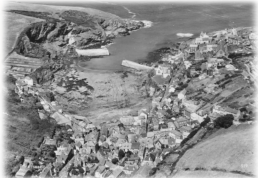
This picture taken in about 1960 shows a natural harbour facing the north west and open to the Atlantic weather. The Breakwaters were built at the end of the 1920s, but the Western Breakwater was built too far in because of financial reasons. The harbour has always been difficult to work. Note how the older portion of the village is condensed in a small area.
