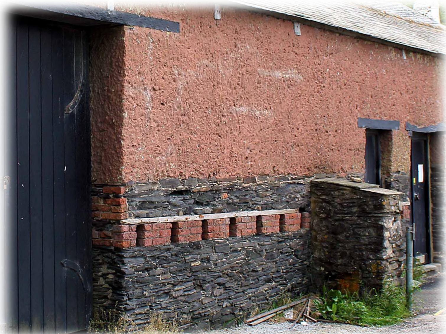
Socket holes in the wall of the Union Cellar, Port Gaverne
