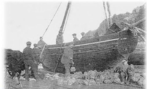
The Boy Fletch, a Provis family boat loading herring nets into the boat. The man holding the cork in the centre of the picture is John Provis, the great-grandfather of the writer. The cork was tied onto the head rope of the net, and more corks are waiting on the sand. Courtesy of Ian Honey, circa 1925
