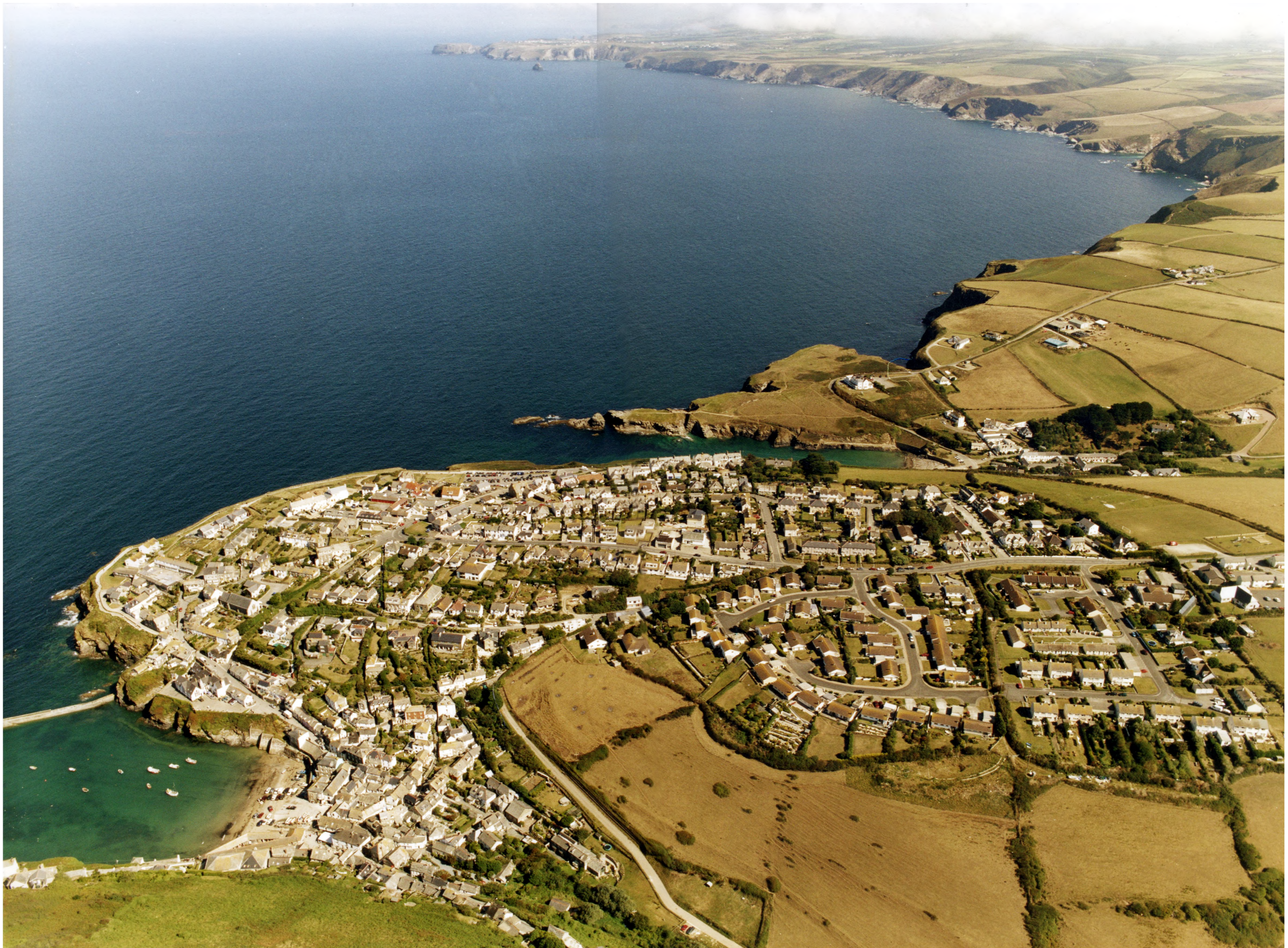
Aerial photograph of Port Isaac, 2001
