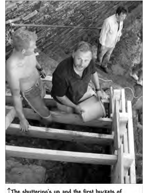
The shuttering's up and the first buckets of concrete are tipped in.
