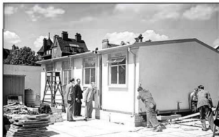
Putting up the four-section AIROH home on prepared foundations in a few hours with just a handful of men
