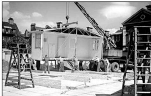
Putting up the four-section AIROH home on prepared foundations in a few hours with just a handful of men
