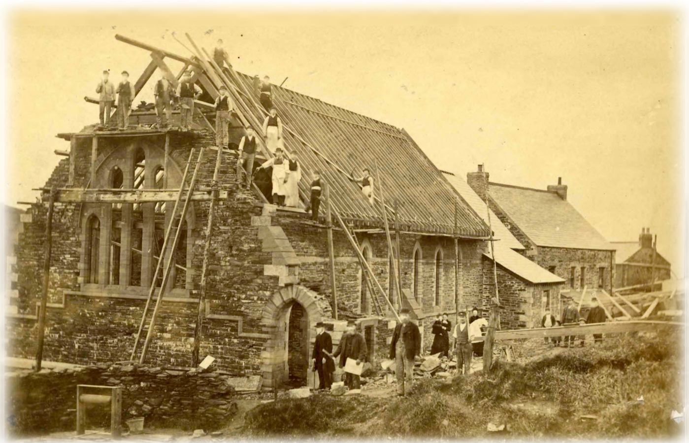
St Peter's Church being built in 1882 - note the five windows at the front that were replaced by just three windows in 1932
