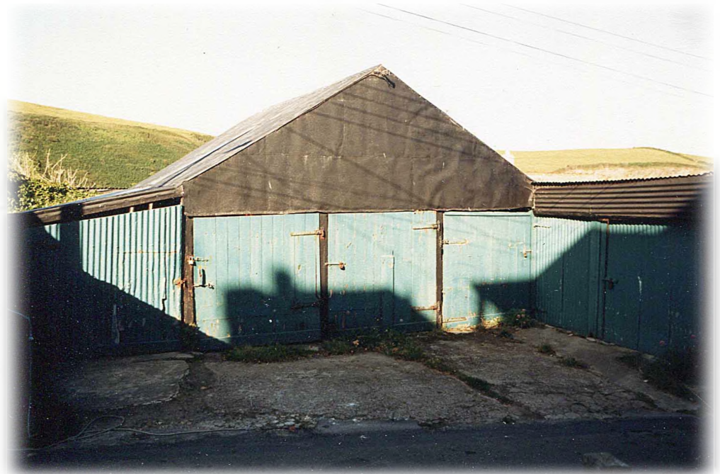
The Old Coal Store before it was renovated by George & Anne Steer
