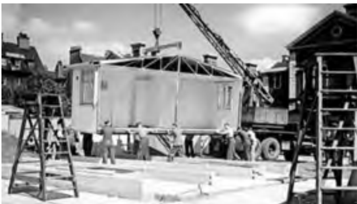
Putting up the four-section AIROH home on prepared foundations in a few hours with just a handful of men
