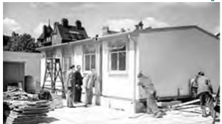
Putting up the four-section AIROH home on prepared foundations in a few hours with just a handful of men
